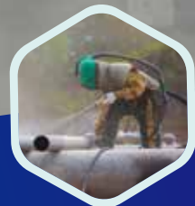
PROTECTIVE COATING BLASTER
